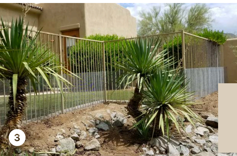
Image 3: Properly installed rattlesnake fencing separating open natural areas from residential activity.
